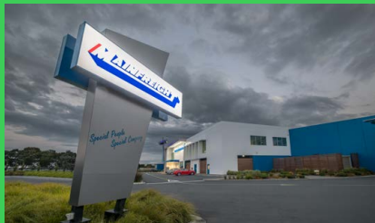
Realizing a bold vision of a modern data center
